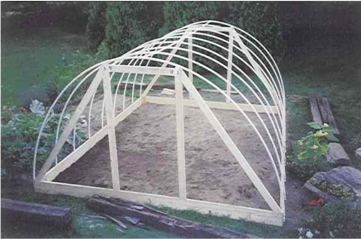
Hoops and sides are in place
