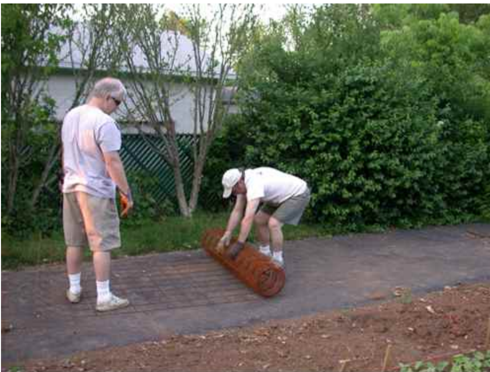
Unrolling the concrete mesh
