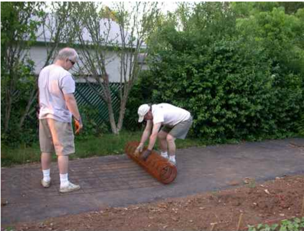
Unrolling the concrete mesh
