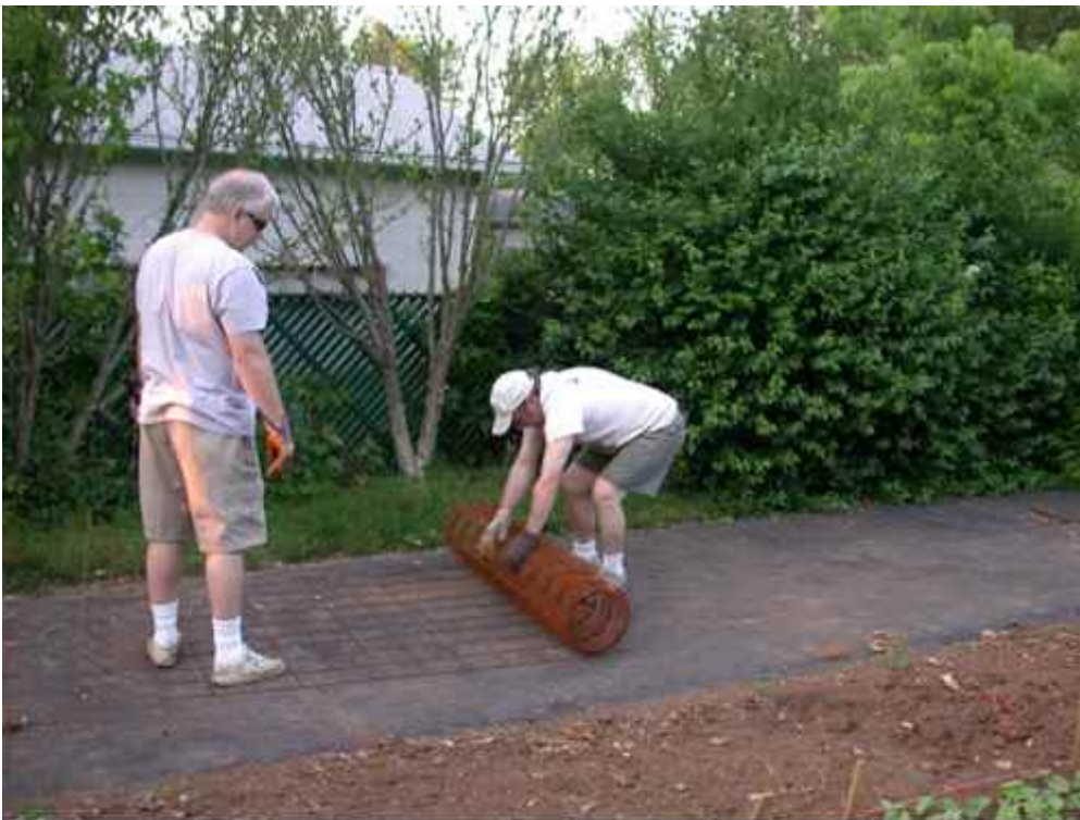
Unrolling the concrete mesh
